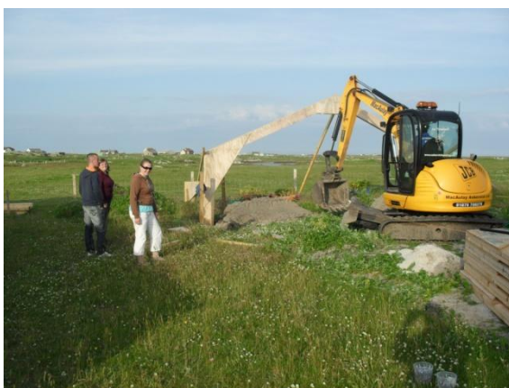
g2 First frame going up on 13th July at 1930 with some of the community greenhouse group looking on.
