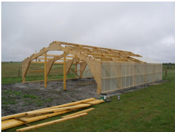
e12 Wall cladding note diagonal bracings
