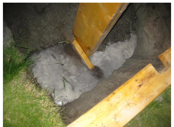
g3 Water in post hole
