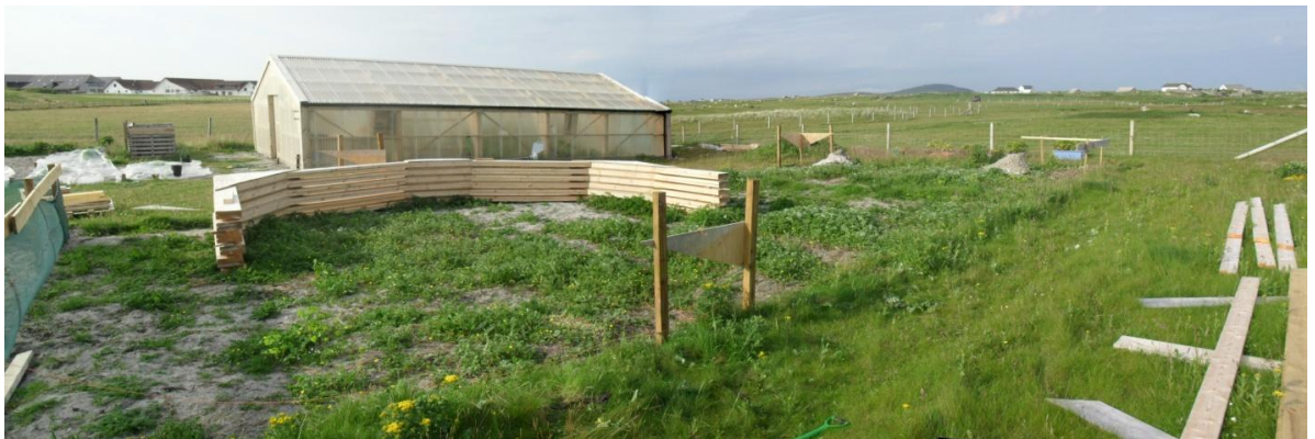
g1 Panoramic view of site prepared for construction
