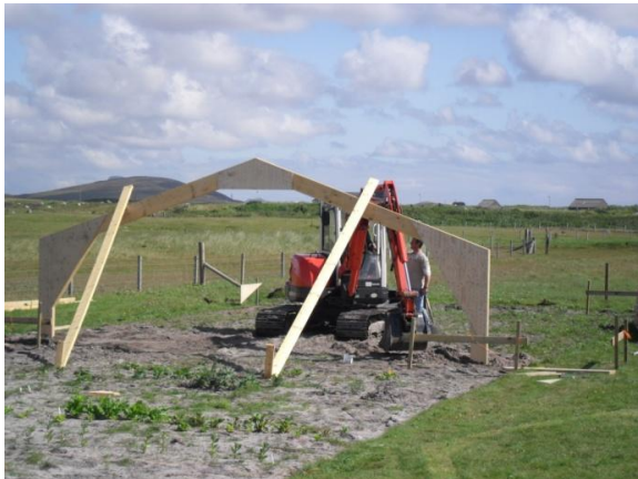
e10 First portal frame in place
