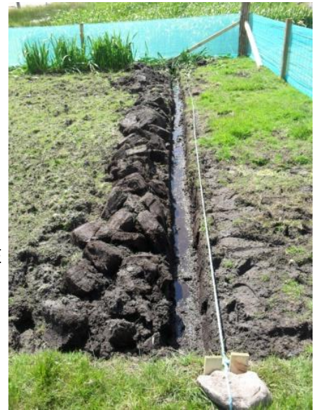
f3 Drainage channel
