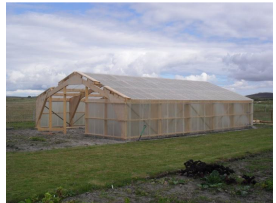
13 Cladding nearly complete
