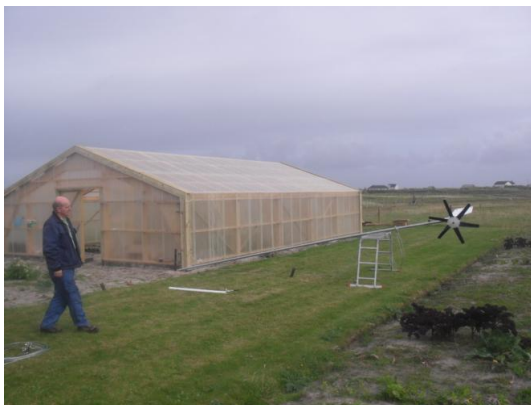
e20 Installation in progress
