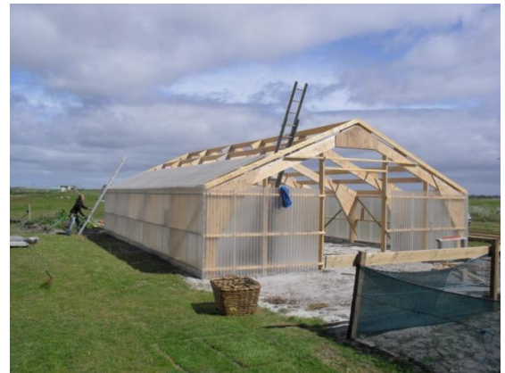
g5 28 th July – sheeting going on
