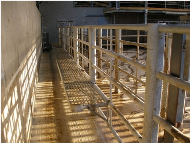
Figure 3 - Raised walkway on race
