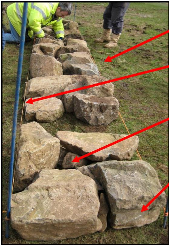
The foundation stones are placed directly on the ground.
